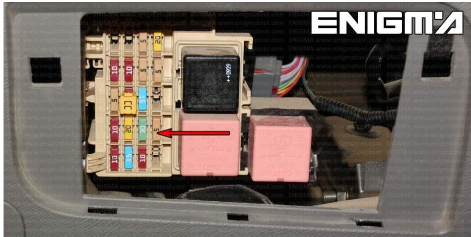
PHOTO 2: Remove the fuse shown on photo above.
